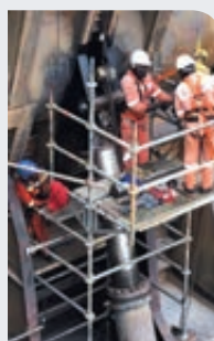
Replacement of the joint of the valve of Channel 2
