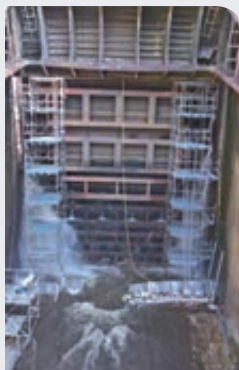
Sluice gate in closed position with significant leakages
