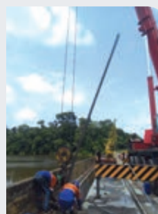
Installation of anchor rods in the body of the dam
