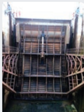
After refurbishment. Sluice gate in closed position. No leakage
